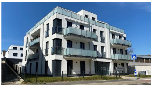
MFH, Kirschenallee (2019, Abriss EFH & Baulücke)
